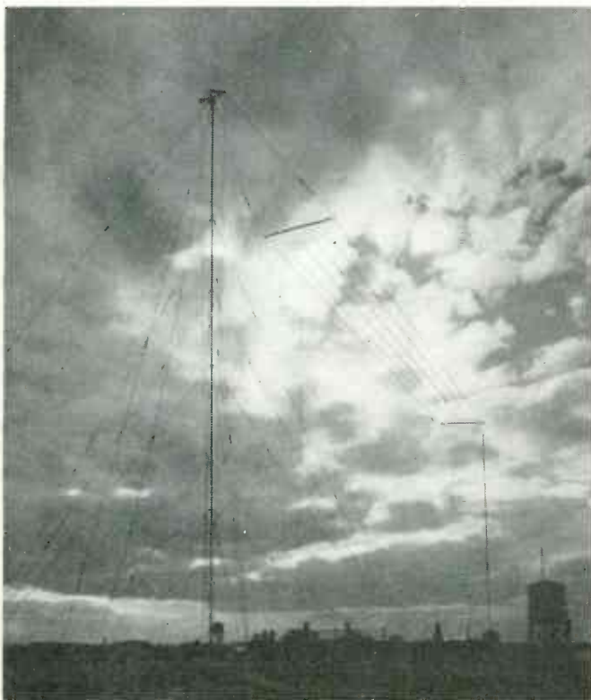
The accompanying photograph illustrates the new antenna system which has just been erected at the WGY broadcasting station. The aerial contrasts greatly with those of our own broadcasting stations which employ a cage type. The flat top aerial seems to be used more in America than here, although many experimenters now employ the flat top for transmission purposes.
