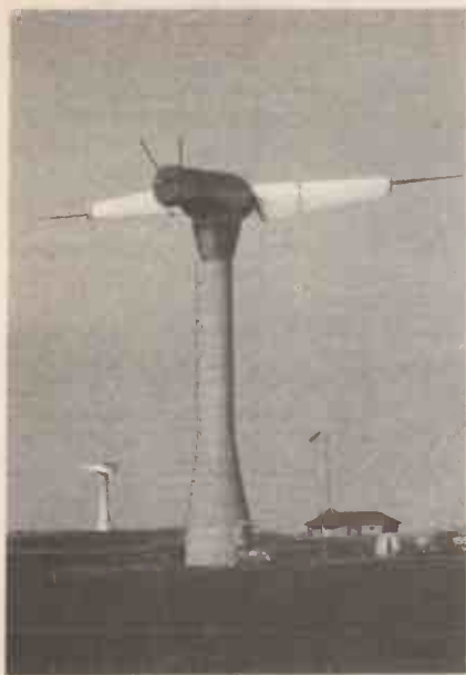
North of Scotland Hydro Electricity Board's 3MW wind turbine at Burgar Hill, Orkney. At 45 metres tall it is one of the largest turbines in the world. It has variable pitch tips and rotates at 34 r.p.m. (Michael Marten/Science Photo Library).
