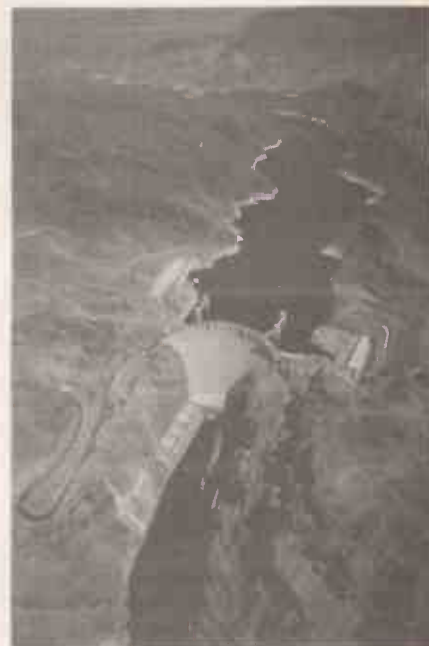
Hoover Dam across the Colorado river, completed in 1936. It is 1,244 feet long and 726 feet high making it the highest dam in the USA. The hydro-electric power station has a generating capacity of 1,000MW from its 18 generators. The reservoir stores 30 million acre-feet of water in Lake Mead which extends 115 miles up the river. (Lowell Georgia/Science Photo Library)
