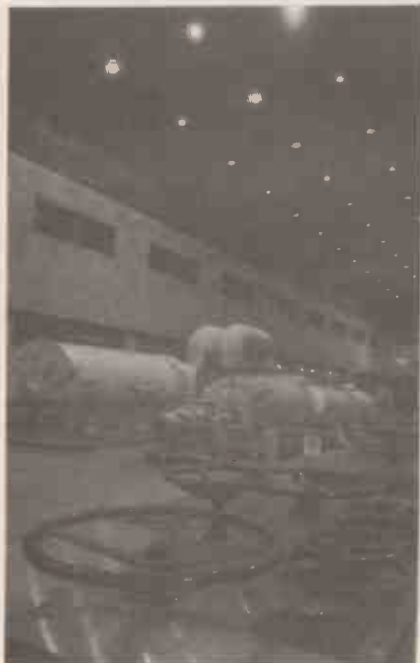
Battersea Power Station showing the main turbine hall. (Sinclair Stammers/Science Photo Library)
