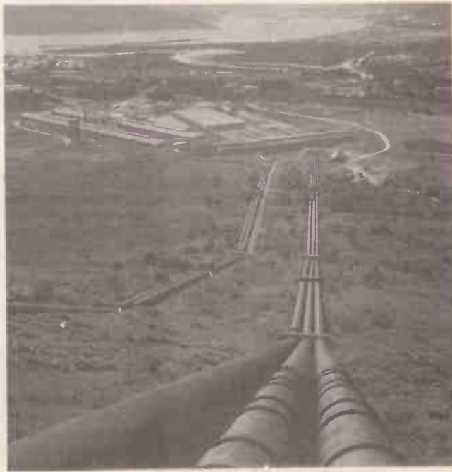
Pipes leading to a hydro-electric power station at the Alcan aluminium works, Fort William, Scotland. (Martin Bond/Science Photo Library)
