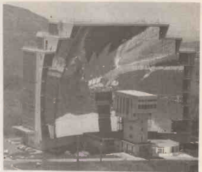
The parabolic reflector at Odeillo-Font-Romeau solar power station composed of 9,500 mirrors. The furnace is capable of generating 1MW of thermal power. (Tony Craddock/Science Photo Library)
