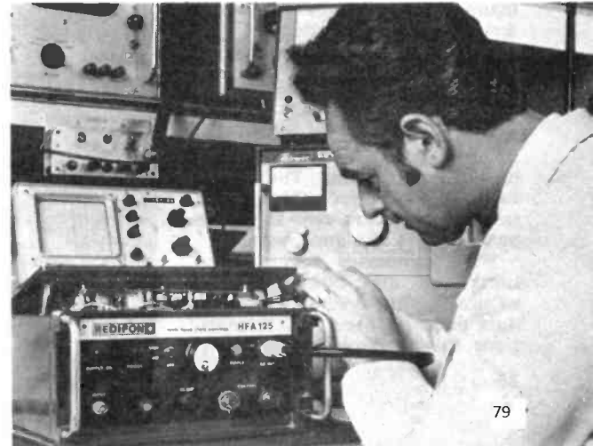
Adjusting an HFA 125 100W solid state HF amplifier, an example of third-generation solid state equipment designed for the military and naval markets.
