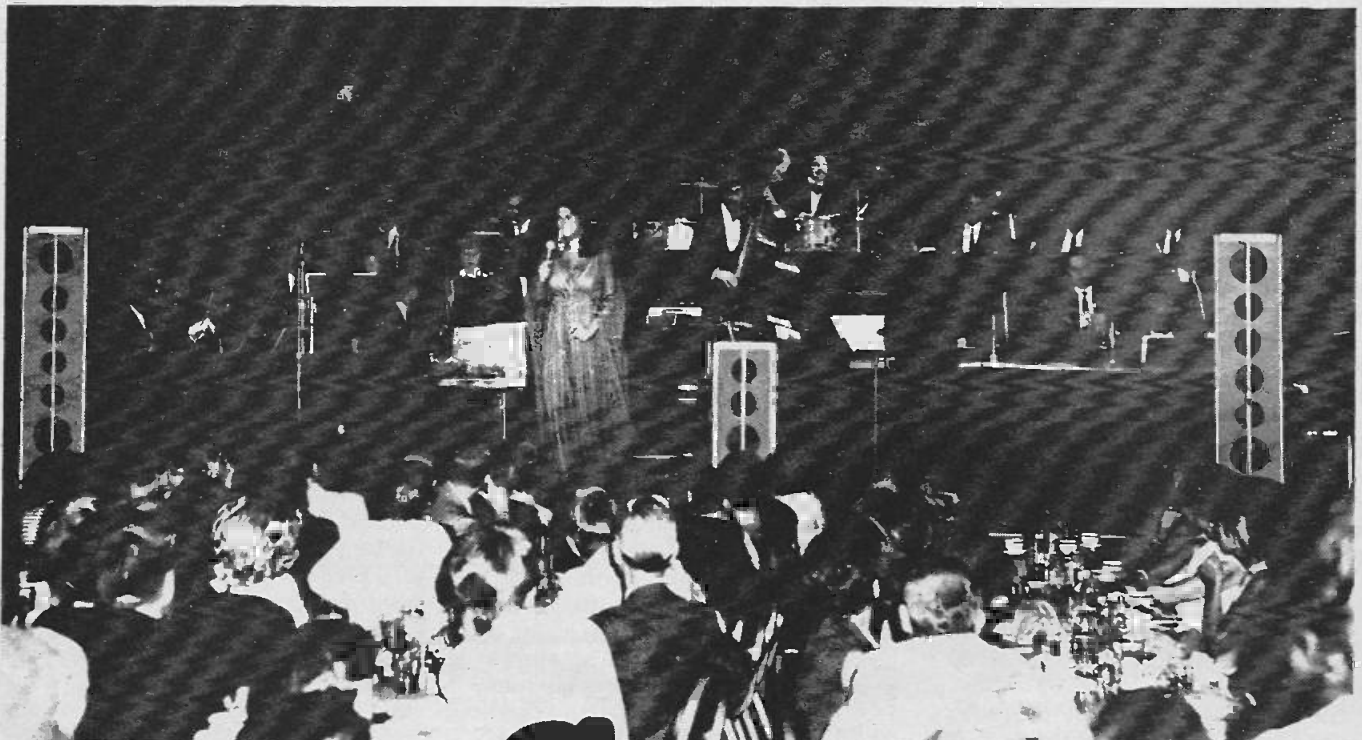
The "small" centre speaker enables the entertainer to hear herself. It also provides sound fill for the first four rows of the audience. The column speakers located at the sides of the stage provide source-oriented sound covering entire auditorium.
