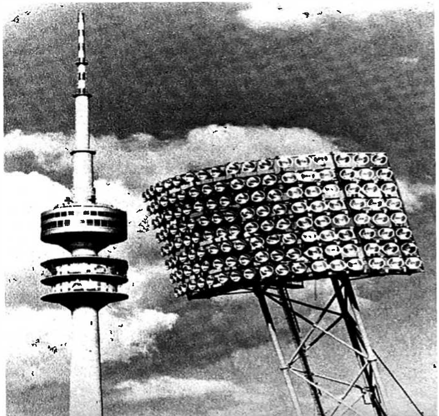
A total of 550 floodlight projectors are used in the main Olympic Stadium. This illustration shows one of the two main towers each with 144 projector units. The total installation draws over 2,000,000 Watts.
