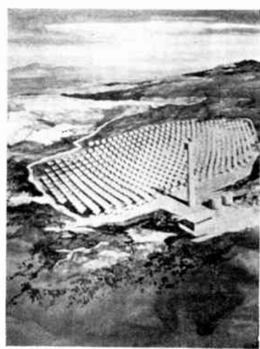
Fig. 2. Artist's impression of the French 2 MW solar power station to be built in Cerdagne in Pyrénées-Orientales. The boiler is mounted on top of the 80m tower and faces north. (Centre National de la Recherche Scientifique).
