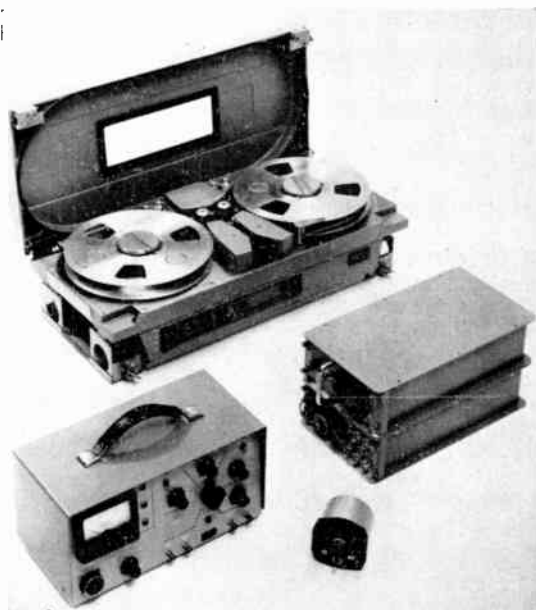
Fig. 6. 7-channel airborne recorder with remote control and test equipment.
