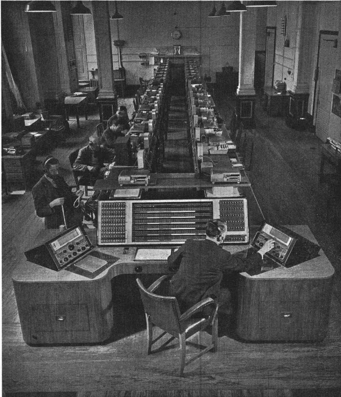
Fig. 7 — Part of the main listening room at Caversham showing monitoring benches and the supervisory console
