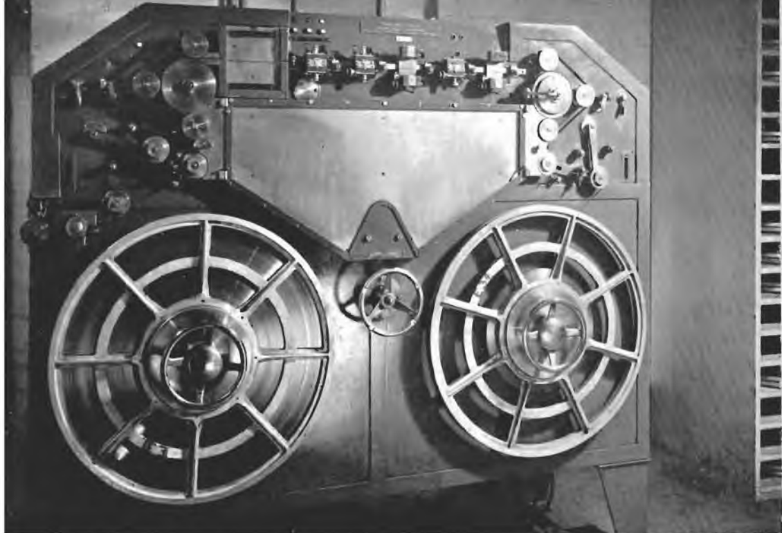
Marconi-Stille steel-tape recording machine
