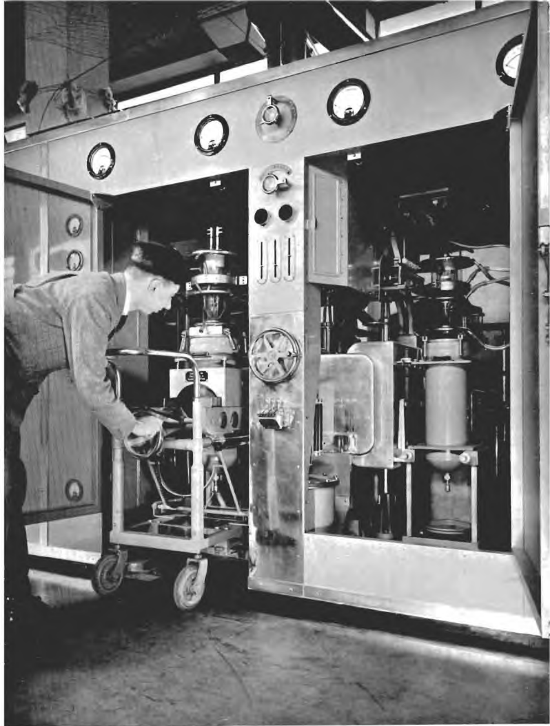
Large water-cooled valve being wheeled into position
