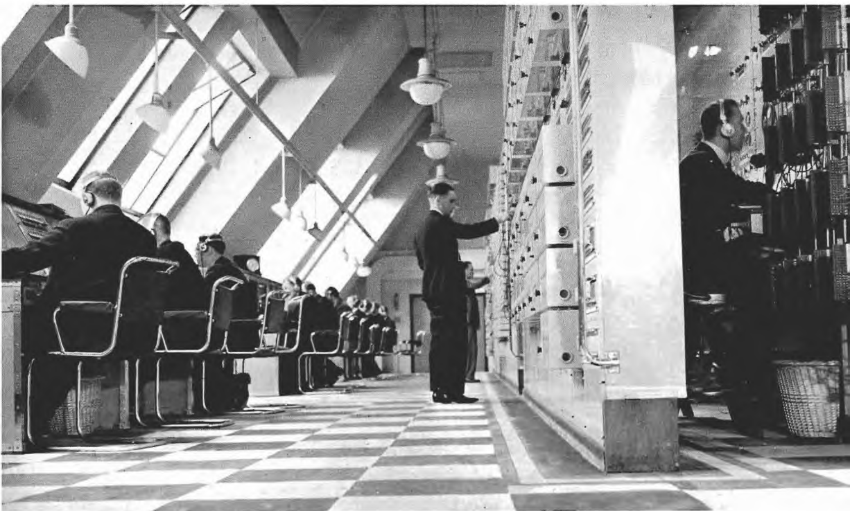
General view of a control room, showing control positions and amplifier bays Plate II
