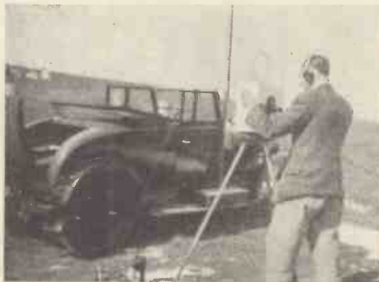
Studying directional effects on a "hot" ultra-short-wave super-het receiver during the tests.
