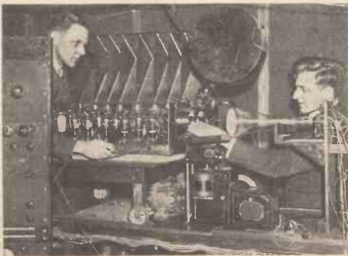
[Wide World photo] Another cathode-ray television system! L. H. Bedford and O. S. Puckle adjusting the new Cossor apparatus, which is claimed to bring the idea of home talking pictures nearer to commercialisation
