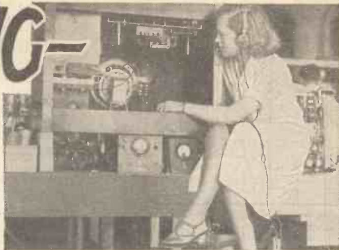
An H.M.V. Super-het Ten Autoradiogram undergoing one of its tests at the Hayes factory. This set now has automatic volume control and a static suppressor
