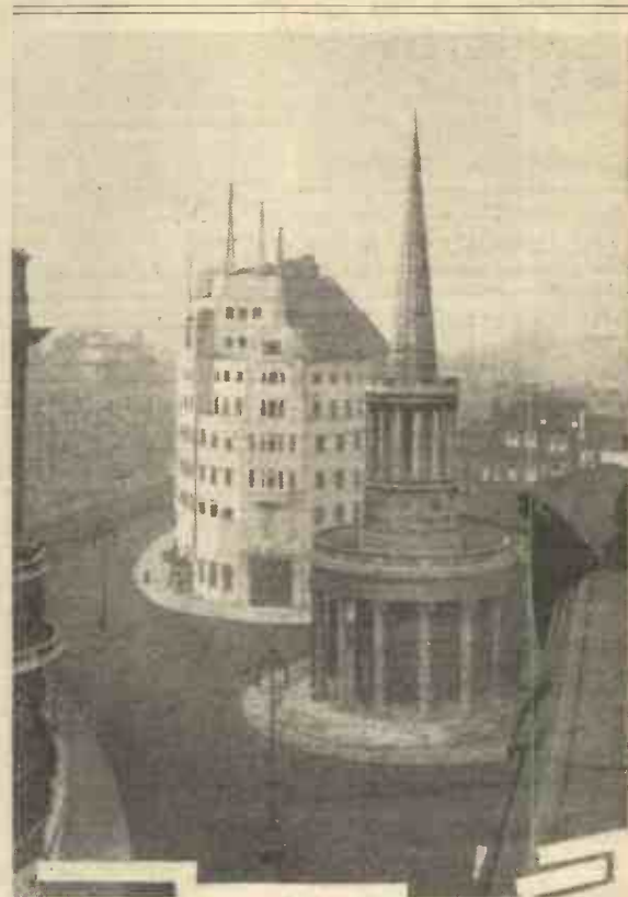
Looking down towards Broadcasting House. The famous All Soul's Church is in the foreground, and the first relayed Service from here was broadcast last week, the Broadcasting House control room being used.
