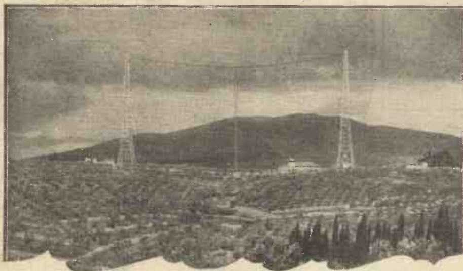
A general view of the site of the Florence station recently opened by the Italian Broadcasting Company. The two masts are each 300 ft. in height, and the transmitting installation consists of a Marconi equipment of 20 kilowatts.
