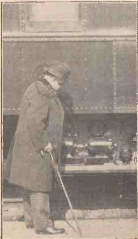
Inspecting the small generators which supply power for the receiver
