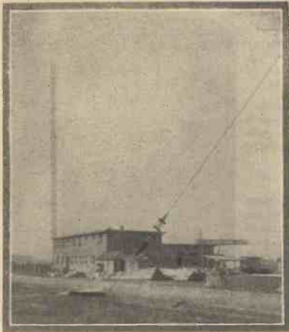
The new Austrian station near Graz
