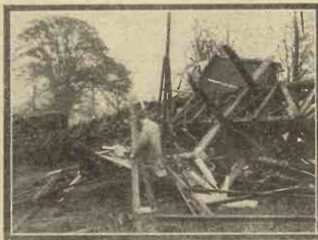
FIRE AT RADIO RESEARCH STATION
