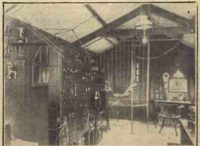
General view of the receiving apparatus at Wroughton
