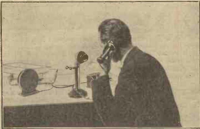
The Telegraphone Records Everything Said and Heard in a Telephone Communication.
