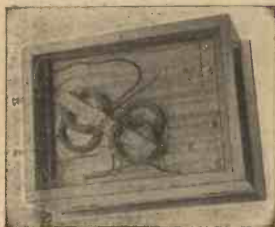
Underneath View of Crystal Receiver.
