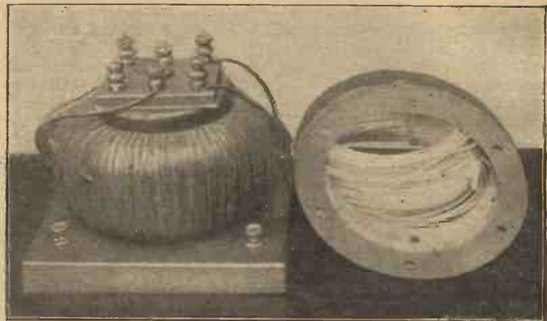
Fig. 2.—Photograph of Complete Transformer and Parts Used for its Construction.
