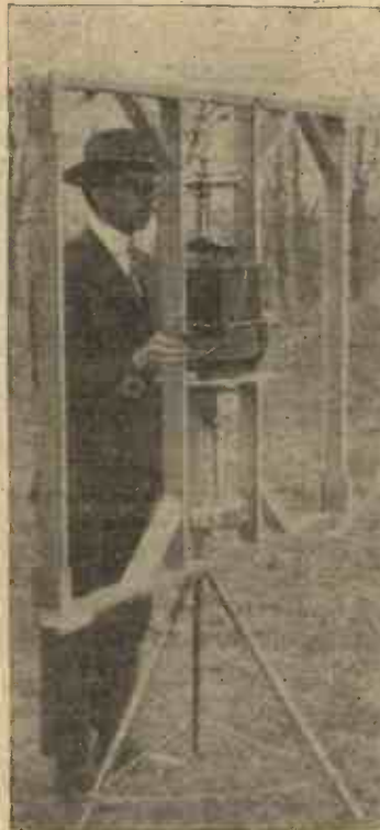
"Blind Spots": Direction-finder Frame Sighting Transmitting Station.
