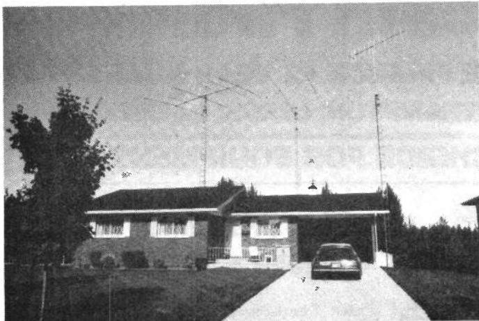
The impressive array of aerials at VE3GCO's QTH in Canada featuring (l to r) a 48ft TH6DXX, a 72ft 204BA and 81ft 402BA and a 14 ele 2m VHF beam
