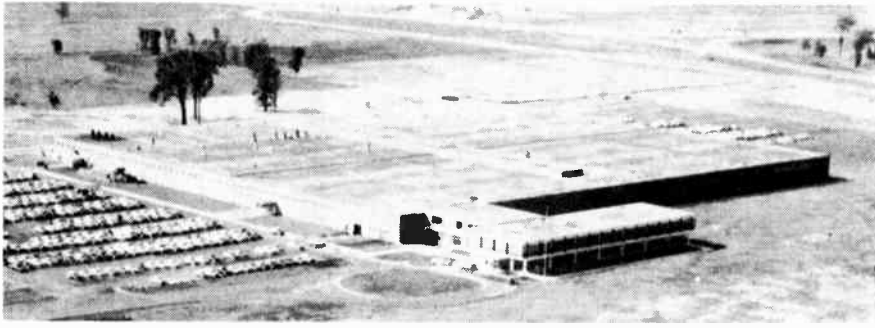
The new London Works of Northern Electric Company Limited which were formally opened on September 30 by Honorable J. P. Robarts, Q.C., M.P.P., Minister of Education for the Province of Ontario. The London Works will be an entirely self-contained manufacturing operation, producing telephone and outside plant apparatus all the way from raw material to the finished product.
