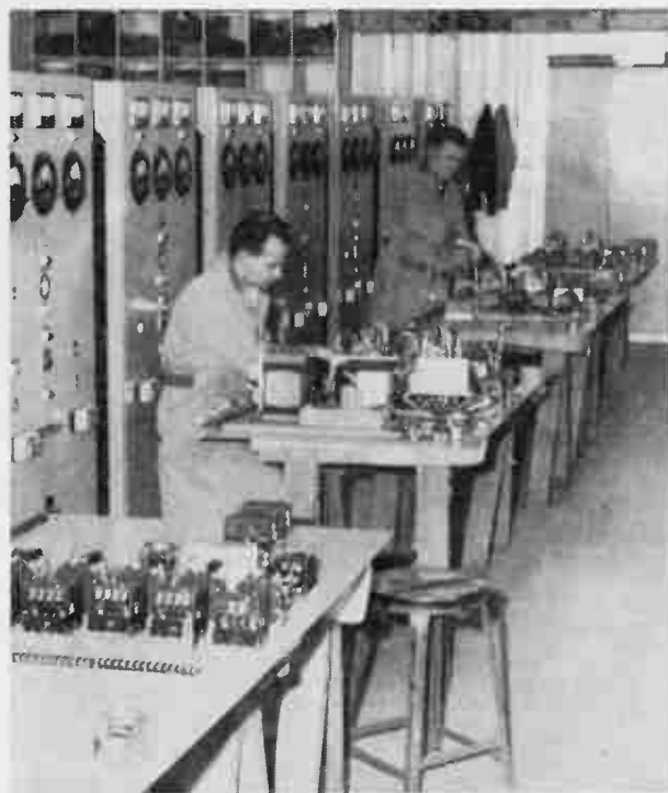
A portion of the control cubicle assembly line at Mechron Engineering Products, Ottawa, Ontario. These cubicles form part of No-Break power plants providing uninterrupted power and supplied by Mechron to the Department of National Defense.
