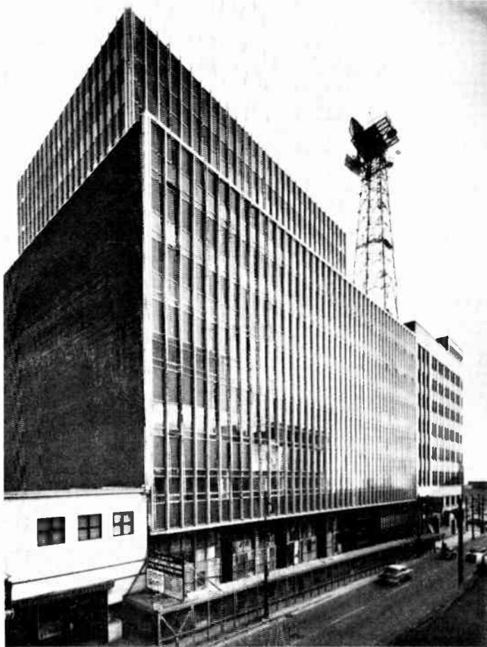
This 12-storey addition to the William Farrell Building in downtown Vancouver will more than double available headquarters space when it is occupied this summer. B.C. Telephone Company departments now housed in 10 different locations will be brought together in the new quarters.
