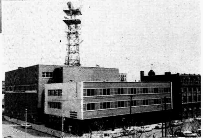
S.G.T.'s 12th Avenue Building, Regina, including the offices and the local, long distance, microwave, TV and distance dialing equipment it houses, is valued at over $10,000,000.
