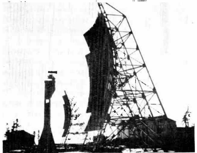
● View of antenna installation in the Quebec-Labrador "tropospheric scatter" radio relay system which will provide commercial long distance telephone service to Goose Bay and the Labrador mining area.
