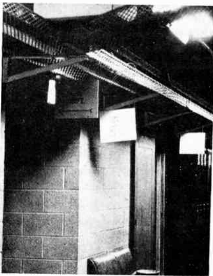
● Left: Cable trough supports thousands of miles of wire and cable throughout the studio. Note the cantilevered supports to which the cable trough is secured. Right: Wires are transferred from cable trough to Cope Cable Ladder to facilitate drop outs to control panels.
