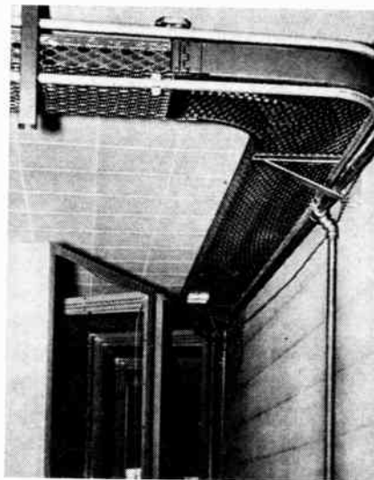
● Left: Close-up of cable ladder. The ease with which cables can be dropped between the rungs reduces installation costs. Right: Cable trough provides a clean, neat installation and at the same time provides access to the cables for re-routing, maintenance, repairs, etc. Note Cope pin-type coupler by which sections are quickly connected. This type of coupler eliminates nuts, bolts, and washers, yet provides rigid support between sections and fittings.
