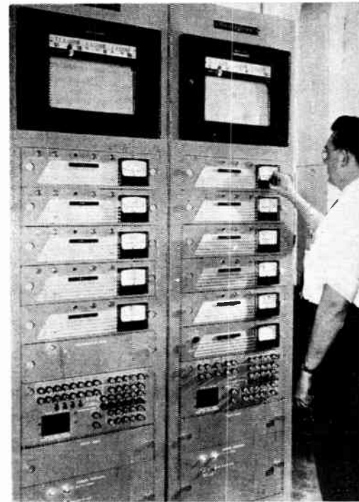
● Westinghouse project engineer is shown adjusting one of the contact meter-relays in a nuclear power plant.
