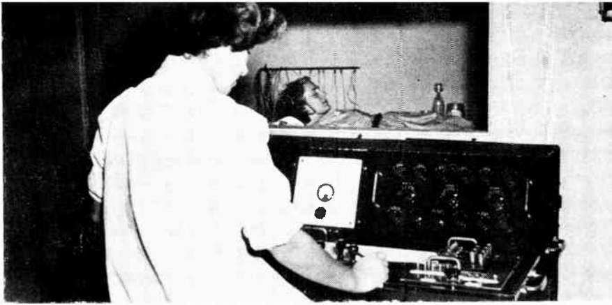
● A special recorder installed in an Electro-Encephalograph at a hospital for nervous diseases.
