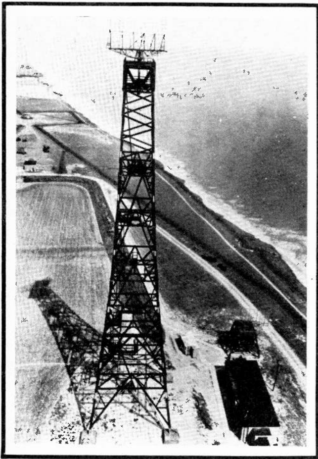
Fig 3. A coastal defence tower. Standing some 360 ft high, the apparatus was used to detect low flying intruding aircraft which were flying too low for normal stations to detect them. Lone raiders often adopted this tactic to reach specified targets, or to make photographic records.
