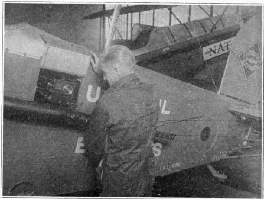
Here is the method of installing the radio receiving sets in N. A. T. mail planes just to the rear of the pilot's cockpit.
