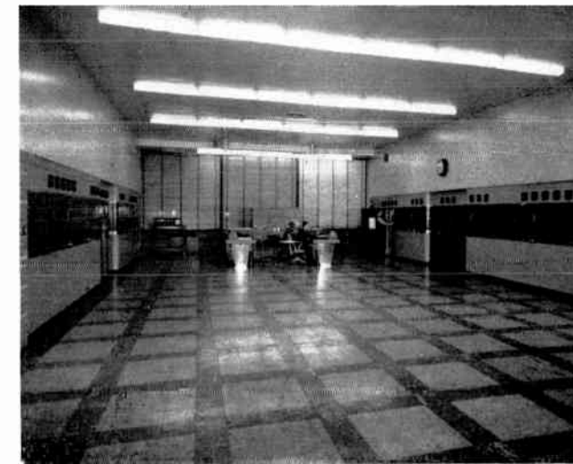
Interior view of short-wave transmitter room shows one 50 Kw. transmitter on each side, with control consoles and speech input equipment between. Operator Bud Fairley tunes up No. 1 transmitter while Russ Walsh at console prepares to feed I.S. program.
