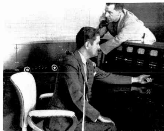
All incoming and outgoing programs are routed to control rooms and various transmitters through Master Control. Operator Russ Walsh has just switched program to short-wave control booth. Operator Reg Howley is talking on order wire line to CP repeater at Moncton, 133 miles distant.
