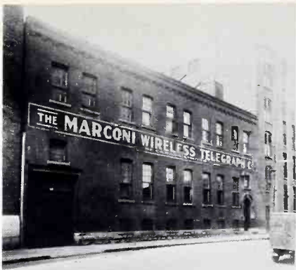
The Marconi factory building on William Street in downtown Montreal. XWA began in the corner on the second floor.
