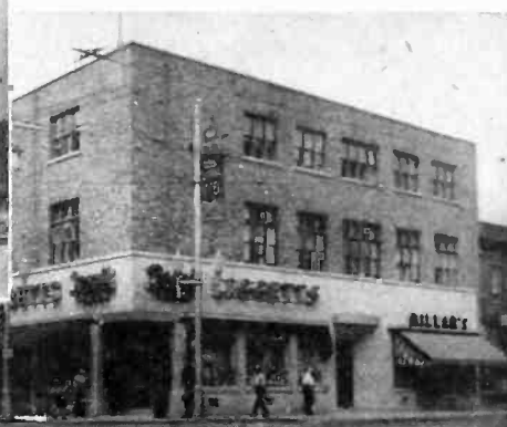
BELOW—The Modern Extension and Front of King George Hotel with New Stores.
