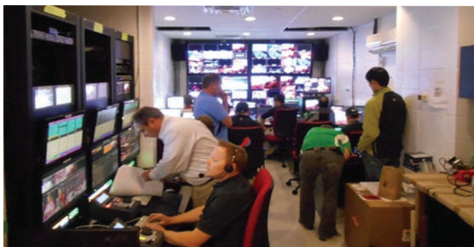
Inside the Saddledome's new broadcast and production control room
