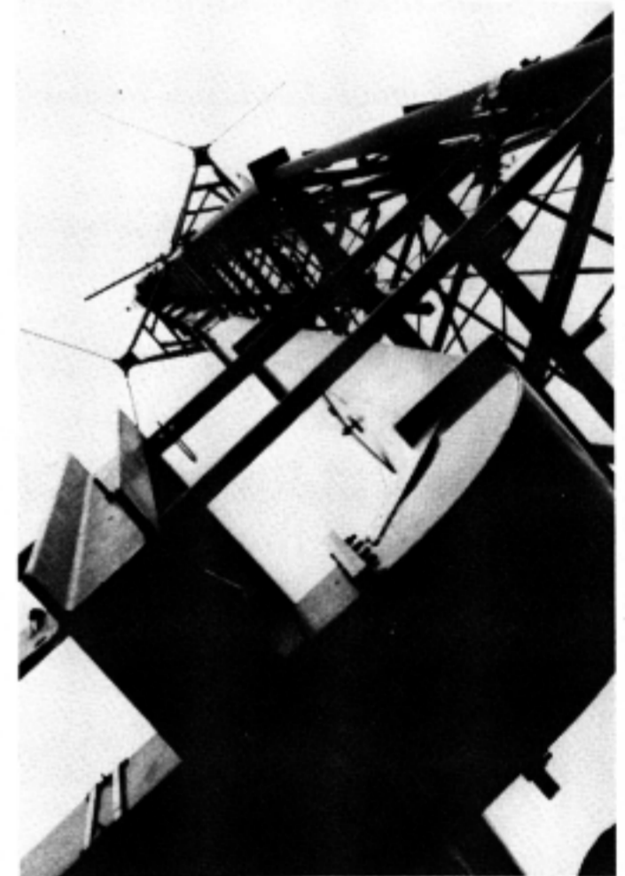
Section of waveguide feed to antenna, showing size in relation to 5-ft tower face.
