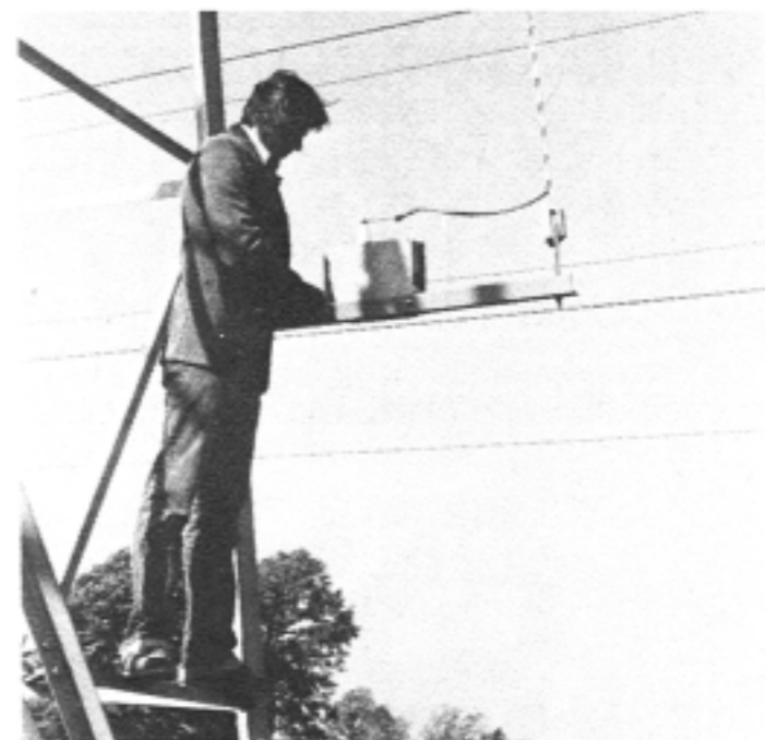
Photo 3: Gary Alford adjusts tuning of revised stub and detuning box assembly.
