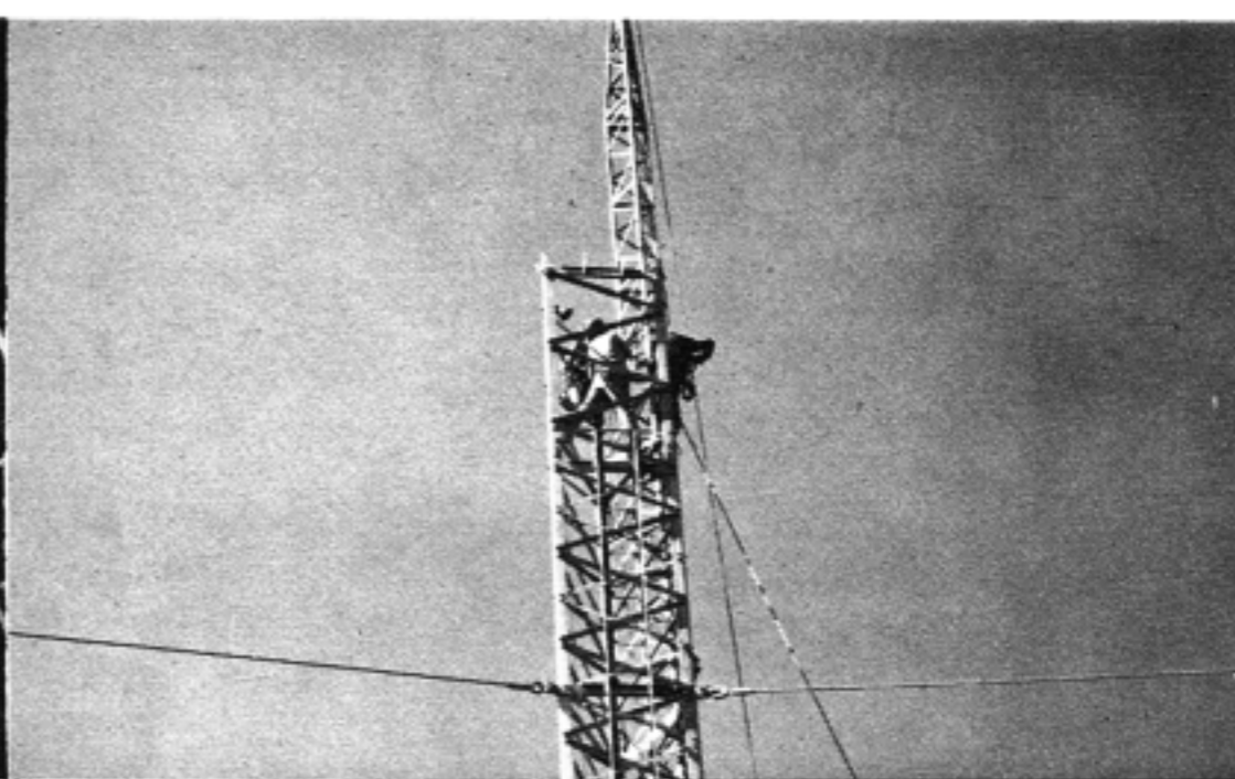
LeBlanc & Royle crew is seen constructing temporary 400-foot tower.
