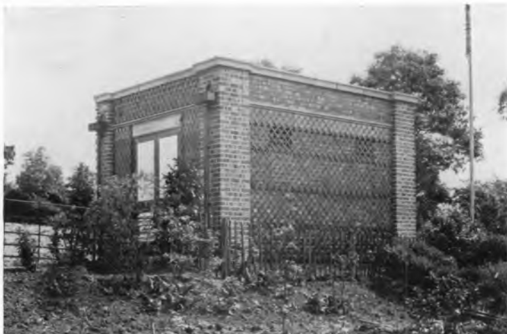
FIG. 35.—A typical form of rectifier sub-station construction which is cheap and yet pleasing to the eye.
