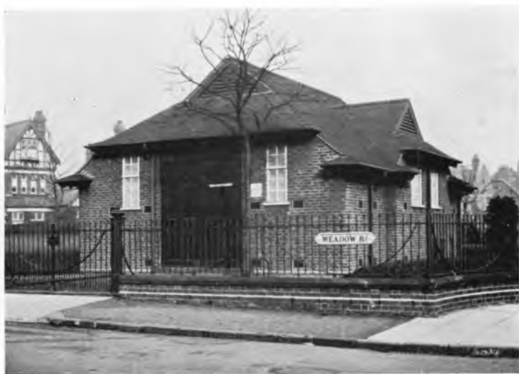
FIG. 36.—A really pleasing type of sub-station architecture.
