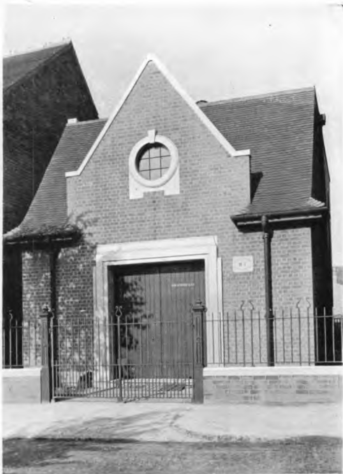
FIG. 39.—Another pleasing type of sub-station architecture.
