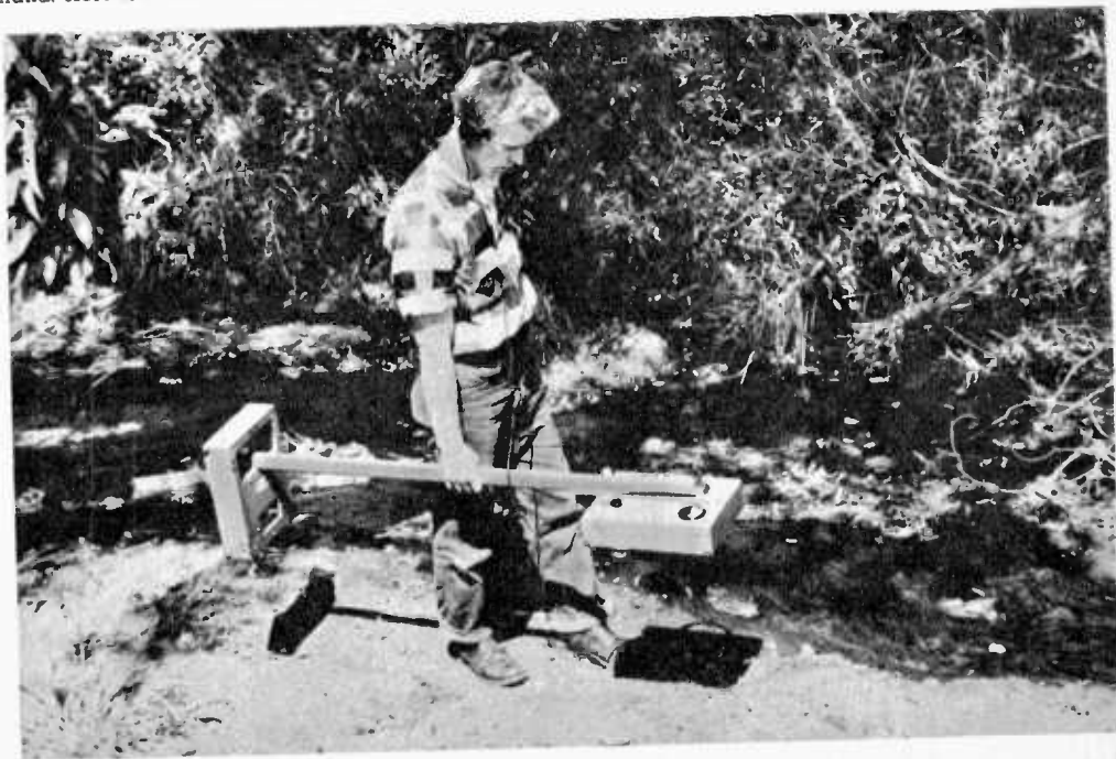
THE FISHER MODEL ME locator (photo above) discloses the presence of an overgrown tower base through its large iron bolts. It's easy to handle.
