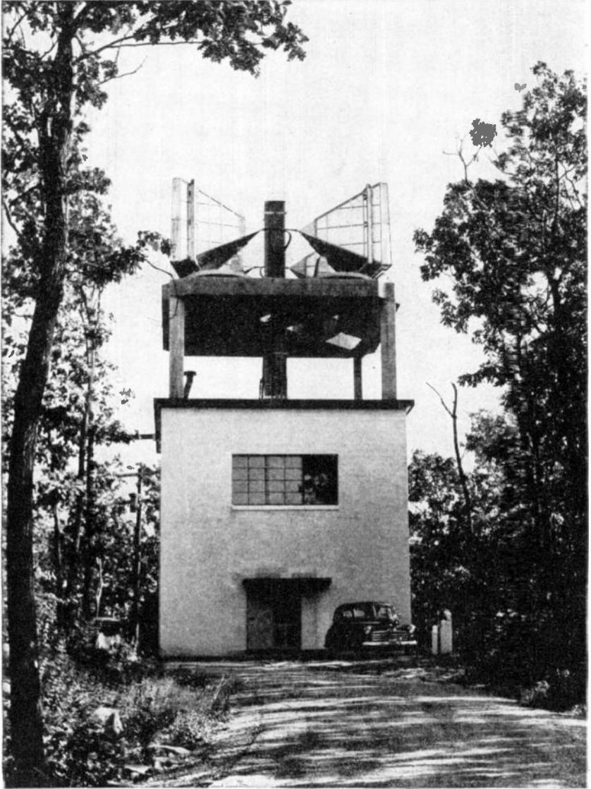
FIG. 125. Typical of the seven intermediate stations on hilltops along the Bell System radio relay route between New York and Boston is the one at Birch Hill, near Patterson, N. Y. Electro-magnetic lenses in the horns seen on the roof receive and beam long distance communication between the two cities.
