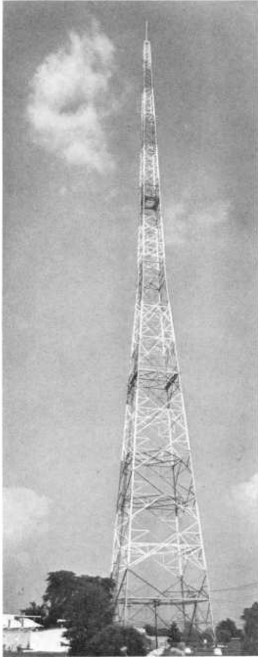
Fig. 1-1. A 500-foot, self-supporting tower. (WLBC-TV, Muncie, Indiana)
