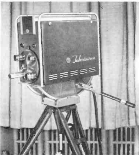
Fig. 3-26. The RCA TK-15A, a studio vidicon camera, uses a 1-inch vidicon tube. (RCA)
