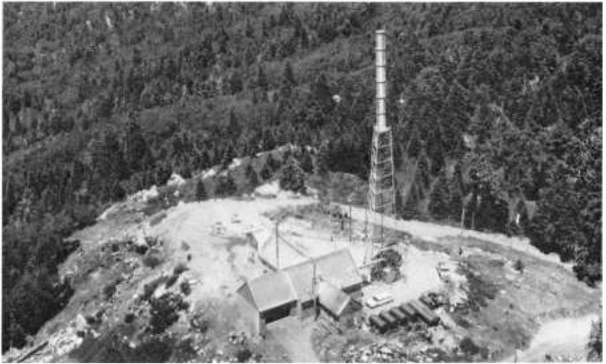
Fig. 2-5. This antenna location is 3697 feet above average terrain at an altitude of 7622 feet above sea level. Used by KERO-TV, Bakersfield, California, the antenna is enclosed in a radome for protection from severe weather. (GE)
