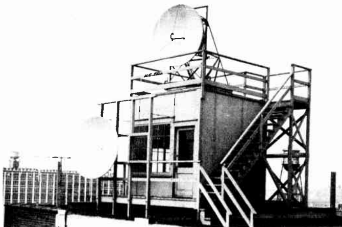
Figure 104. Permanent installation of microwave relay antenna.
