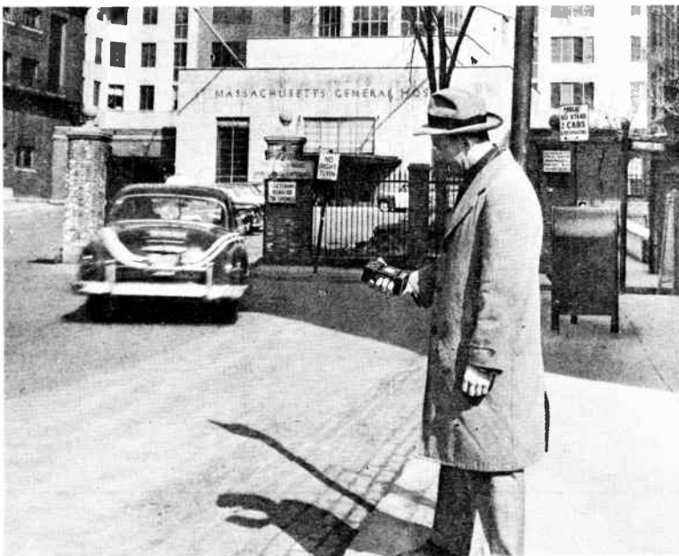
Figure 5-1. The Sound-Survey Meter being used to determine noise levels in a hospital area.
