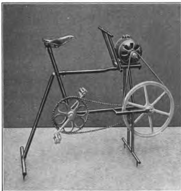
FIG. 50.—Current Generator for Light Portable Stations.
