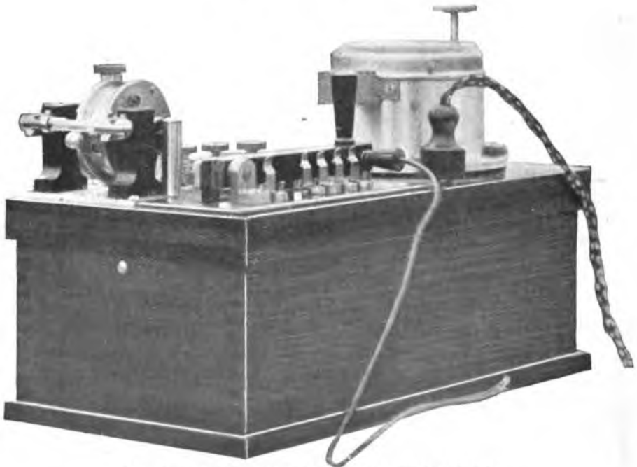
FIG. 63.—Light Receiving Apparatus for Portable Stations.
