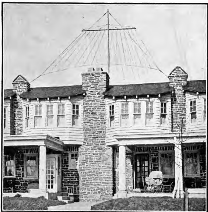
Fig. 62.—Illustrating a high-capacity house-top antenna supported by one mast in which the restricted roof area is used to maximum advantage.
