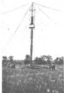
Fig. 313—A Tubular Mast in Early Stages of Construction.
