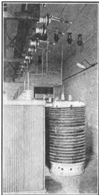
Fig. 307—Bank of High Voltage Trans-formers at Carnarvon Station. Fig. 308—The Switchboard of the New Brunswick High Power Transoceanic Station.
