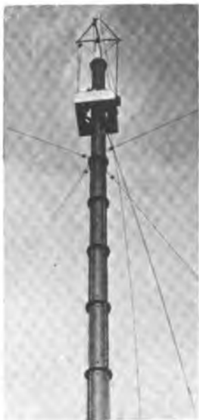
Fig. 314—Showing the Cage and the Top Mast Several Hundred Feet from Earth.
