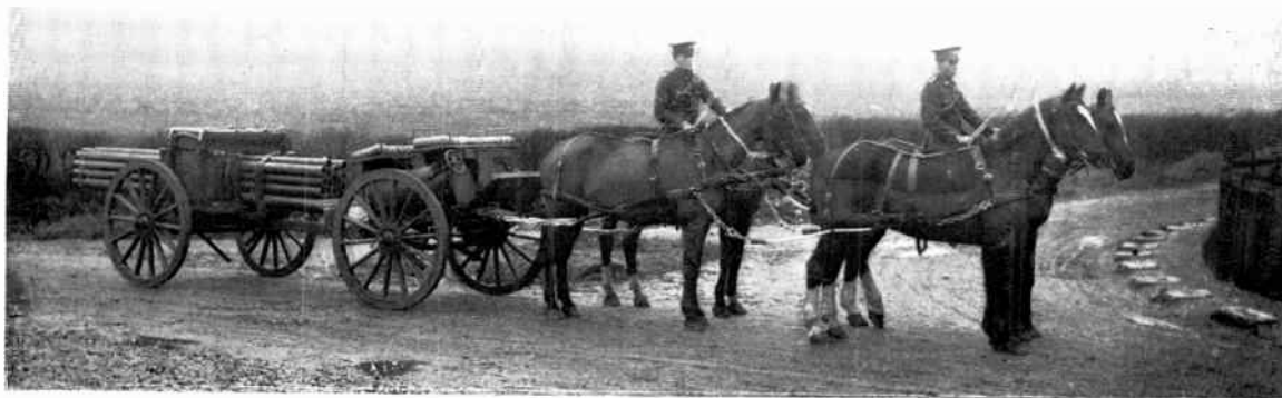
Mast and Supply Cart. Marconi 1½ kw. Field Cart Station.
