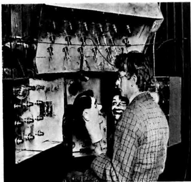
FIG. 91.—Bank of Lamps.
