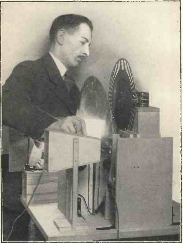
A COMBINED TRANSMITTING AND RECEIVING APPARATUS FOR 30-LINE EXPERIMENTS
